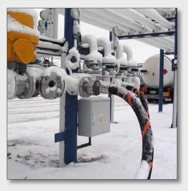
The TODO® Safety Break Away couplings are designed to eliminate spillage and damage associated with drive / pull away incidents.
